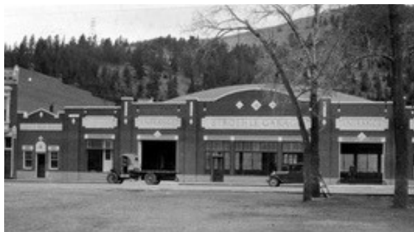
Former parking structure in downtown (now demolished).
