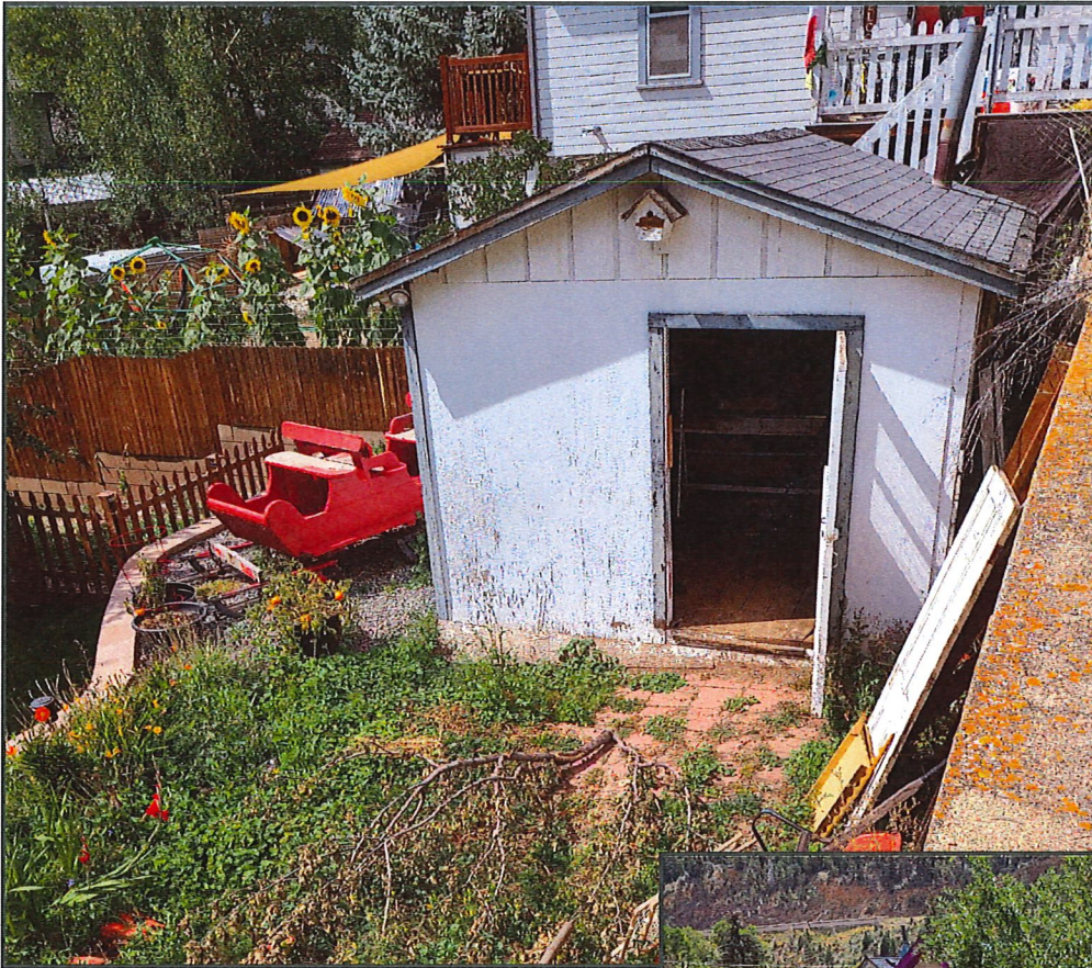
Images of the existing shed from Wall Street.
