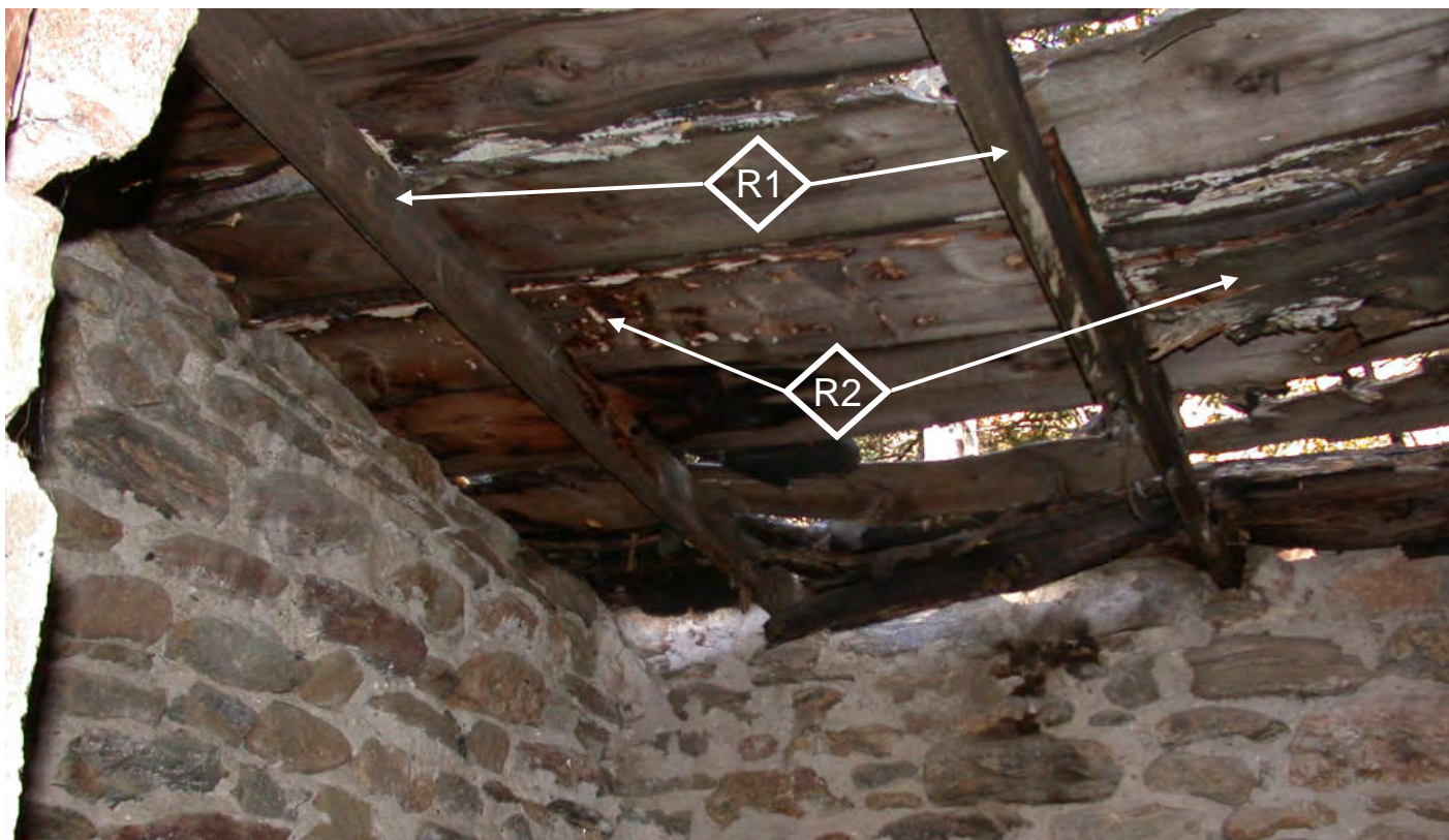
4. Underside of roof – southwest interior corner (September 2011)
