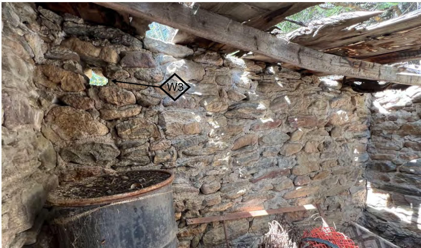
15. South Wall – Interior Face (May 2024)
