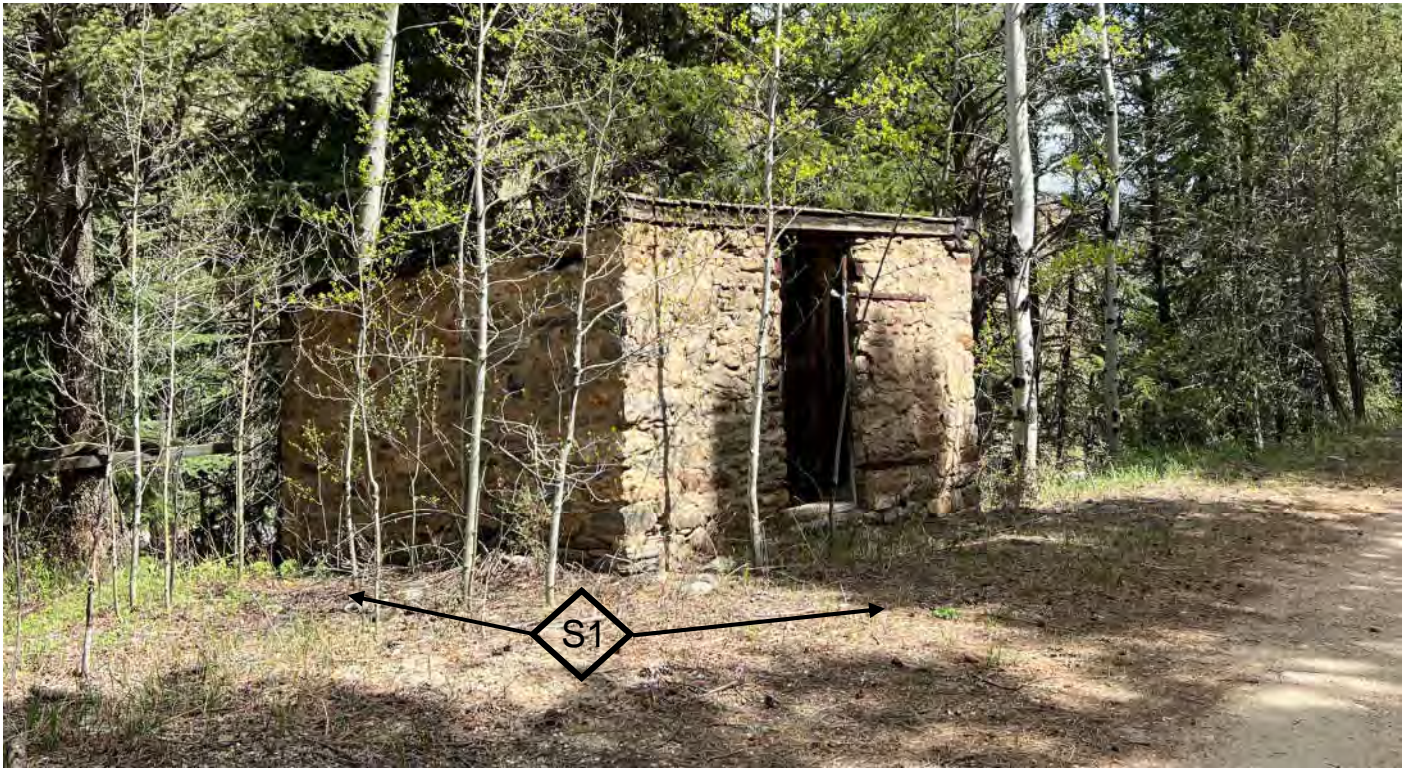
19. View looking northwest at Powder House and site (May 2024)
