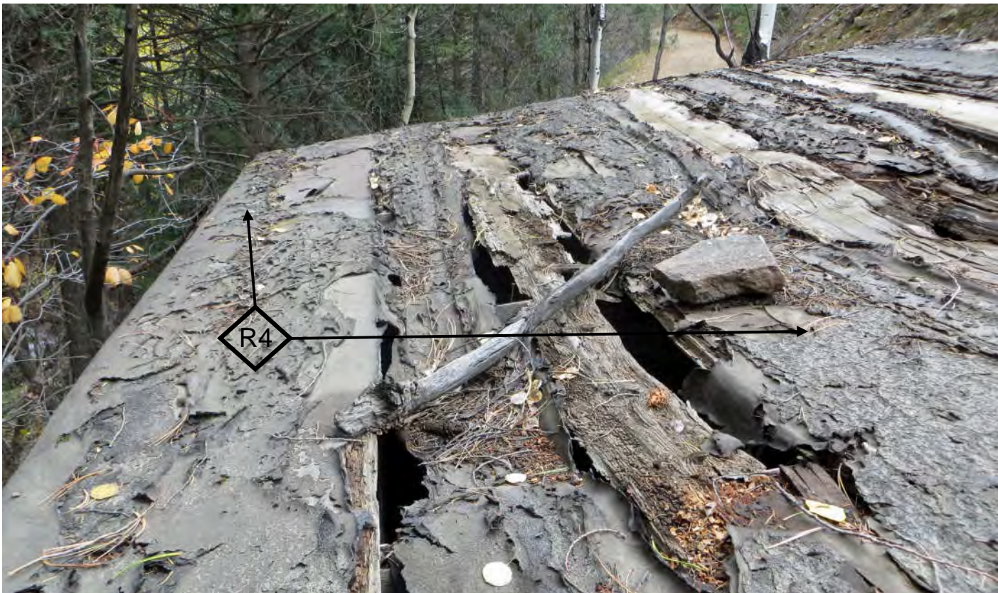
6. Roof looking northwest (October 2013)
