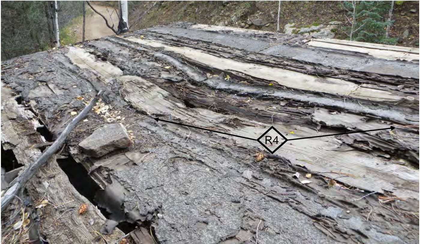
5. Roof looking northeast (October 2013)
