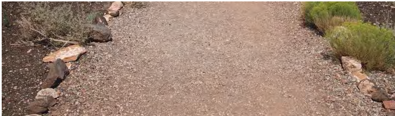
Crusher fines trail lined with native rock; Lomaki Wupatki National Monument, AZ.
