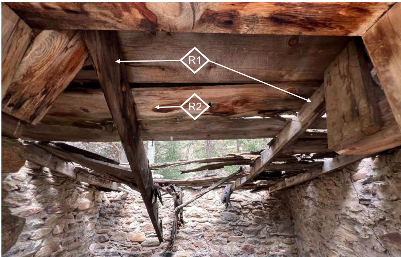
1. Interior west wall and underside of roof (May 2024)
