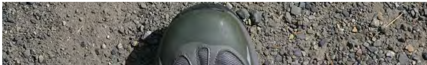
Typical crusher fines surface showing very firm matrix with only a few loose larger rock particles.
