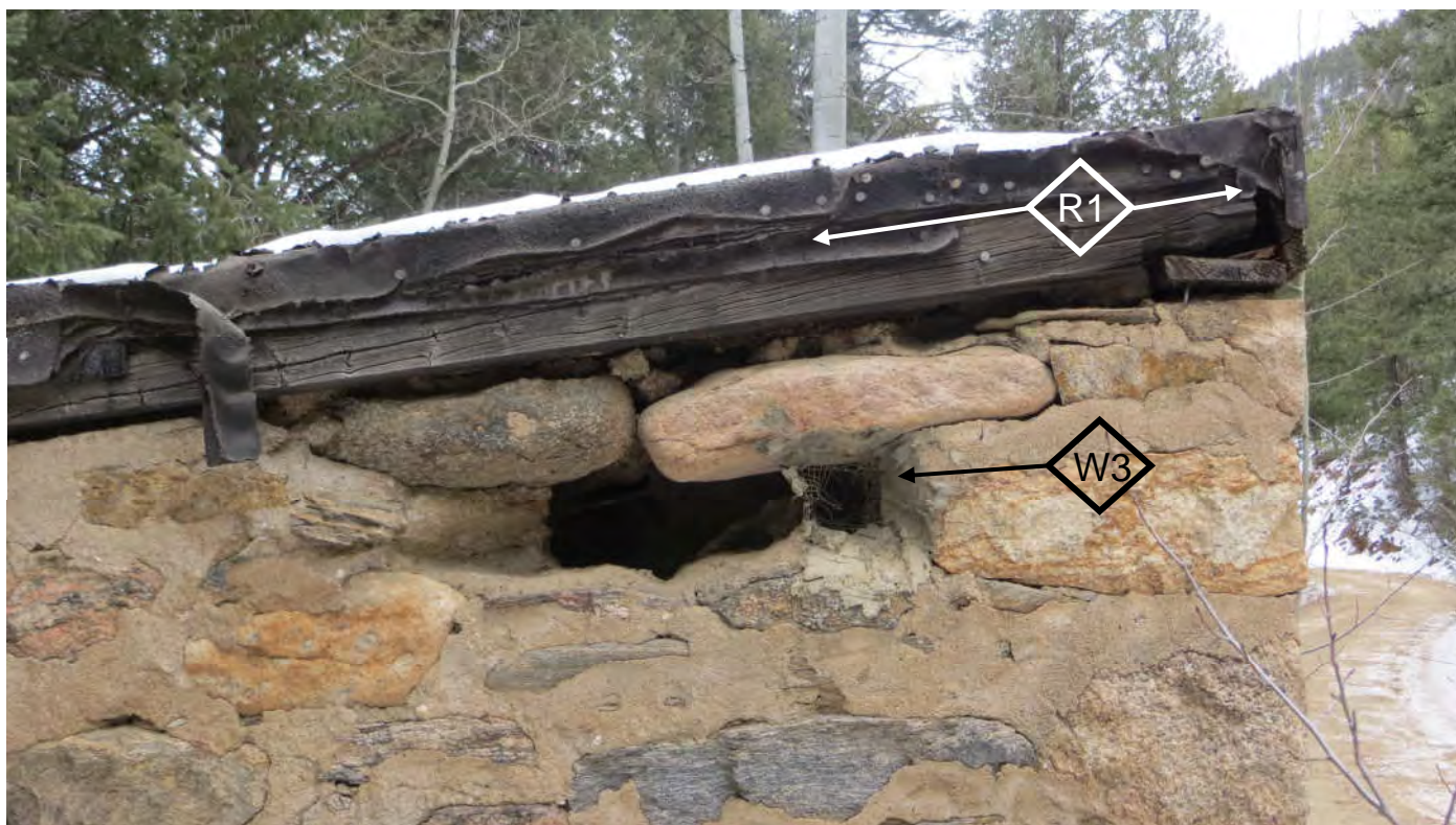
16. Top of South Wall – East End (December 2012)
