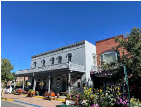
An example of an original porch to be preserved
