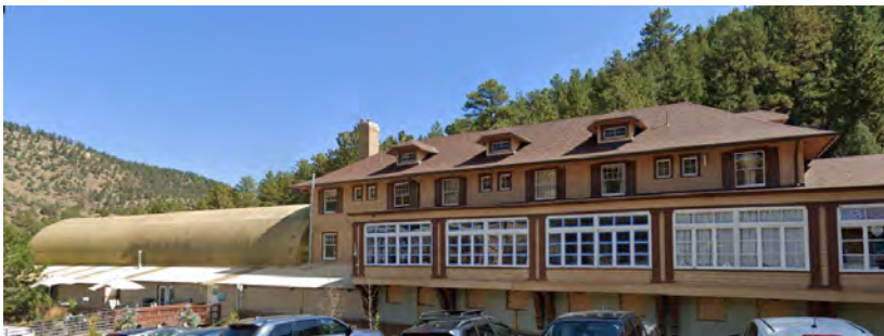
The pool structure at the Indian Hot Springs is an example of a later addition that may have gained significance in its own right.
