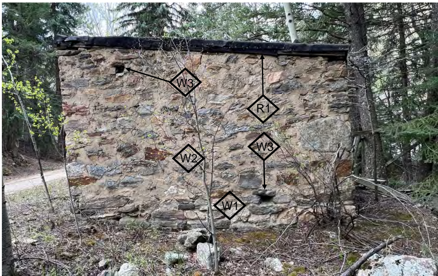
8. North Elevation (May 2024)
