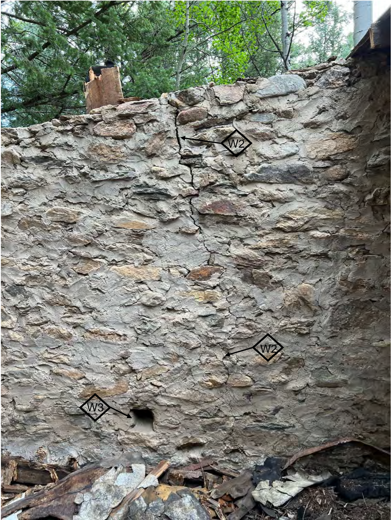
11. North Wall – Interior Face (August 2024)
