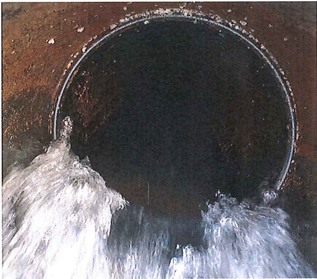
Photo 9 - Looking up outlet pipe
