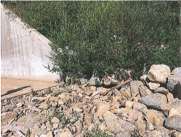
Photo 13 - Left spillway training wall drain outfall location
