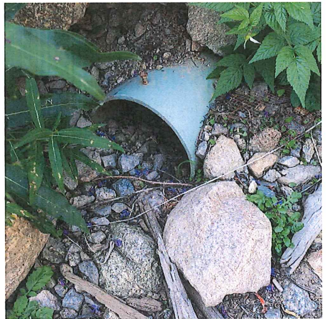
Photo 12 - Right spillway training wall drain outfall
