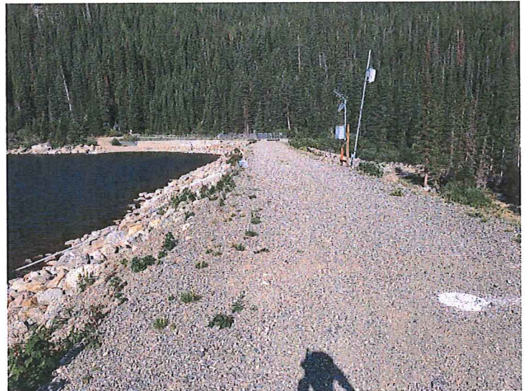
Photo 2 - Crest looking west
