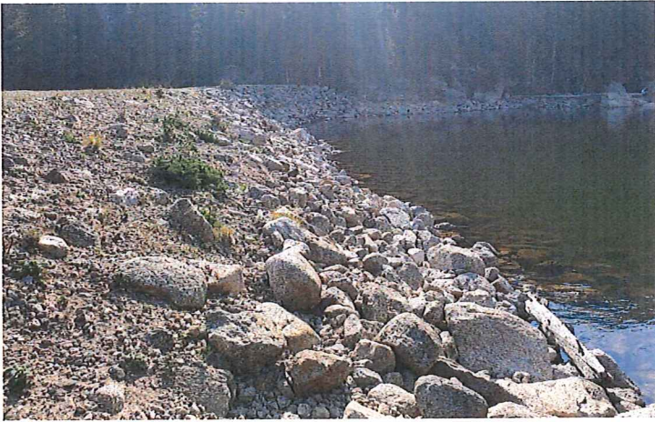
Photo 1 - Upstream slope looking east
