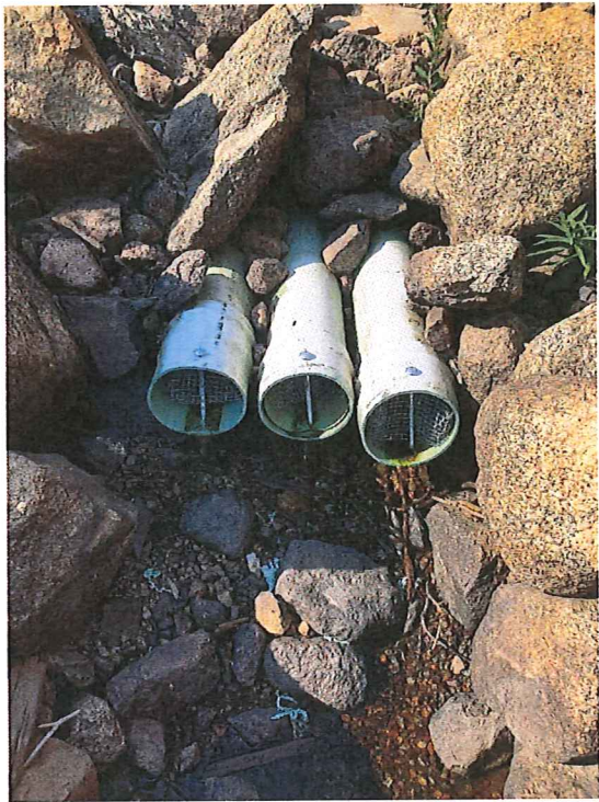
Photo 7 - Toe drain outfall (left) and spillway underdrains
