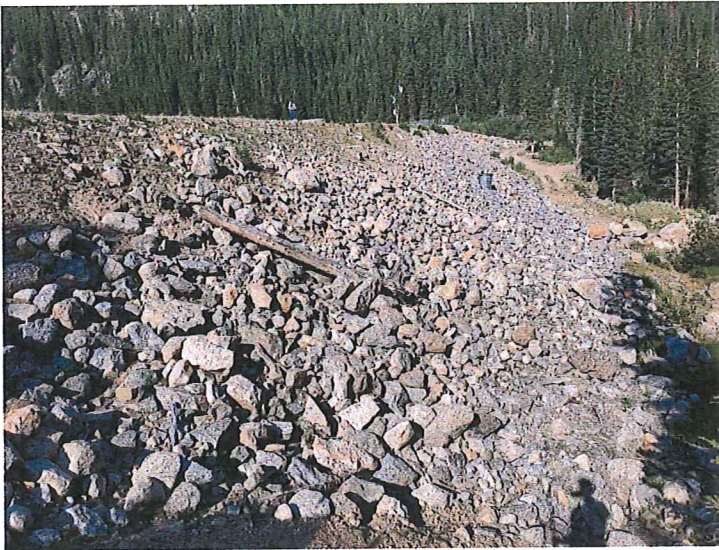
Photo 3 - Downstream slope looking west
