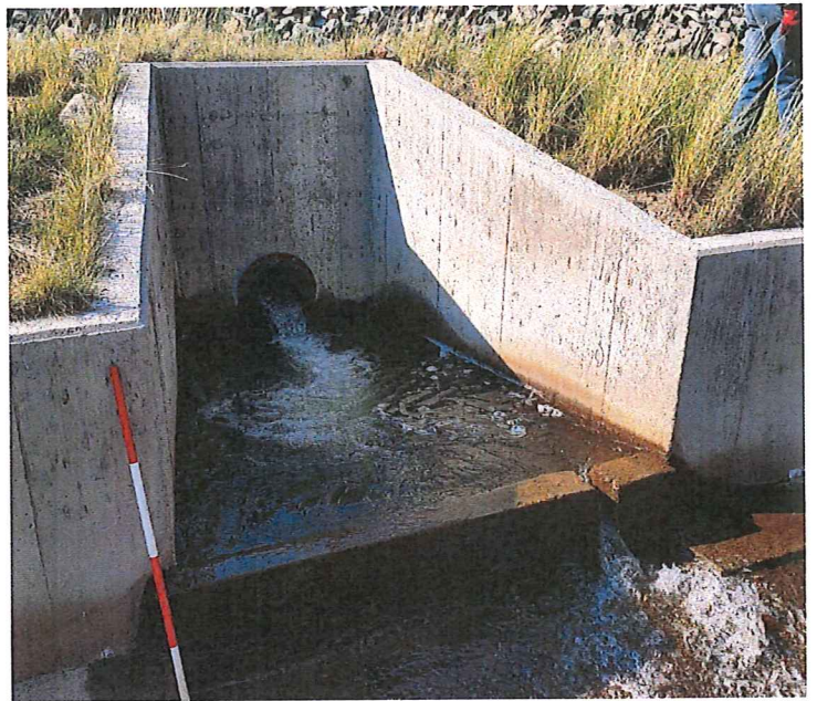
Photo 8 - Outlet outfall structure
