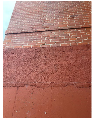
An example of treatment that should be removed to reveal the original finish
