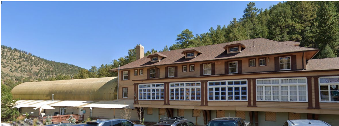
The pool structure at the Indian Hot Springs is an example of a later addition that may have gained significance in its own right.
