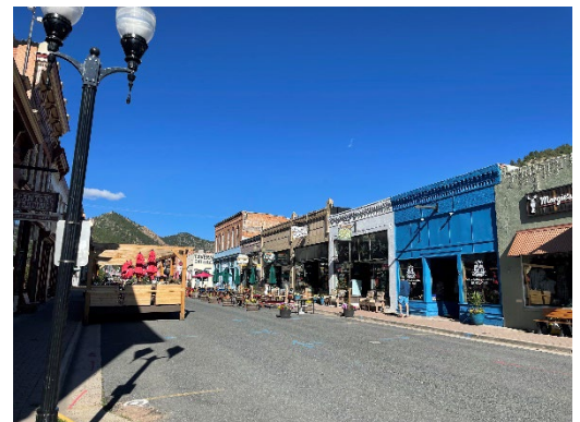
While not perfect, the cornice and clerestory alignment are largely maintained in the District.
