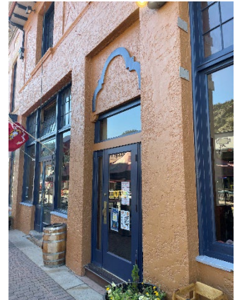
An example of stucco that has taken on historic significance
