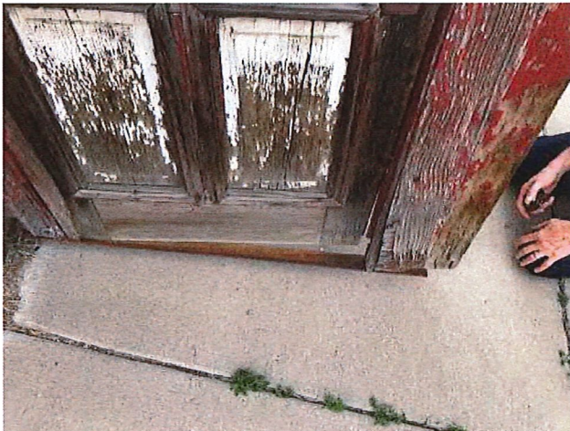
Photo 5 (Above): A steel angle, with the vertical leg cut below the man door, was added to tie the two sides of the door together.
