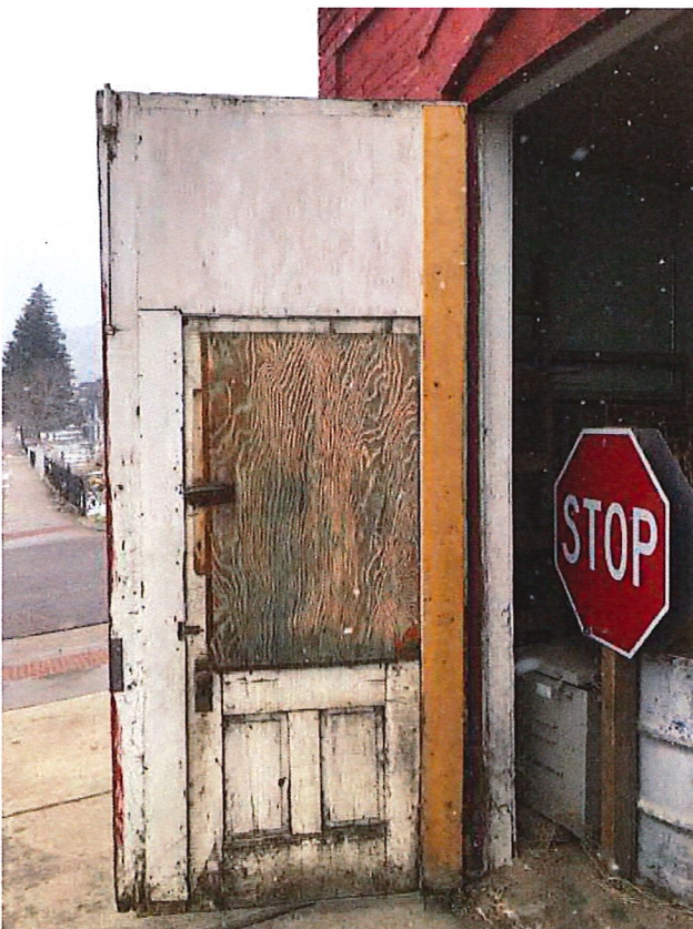
Photo 1: Front elevation of Hose House No. 2 with the addition of the man door in the west leaf.
