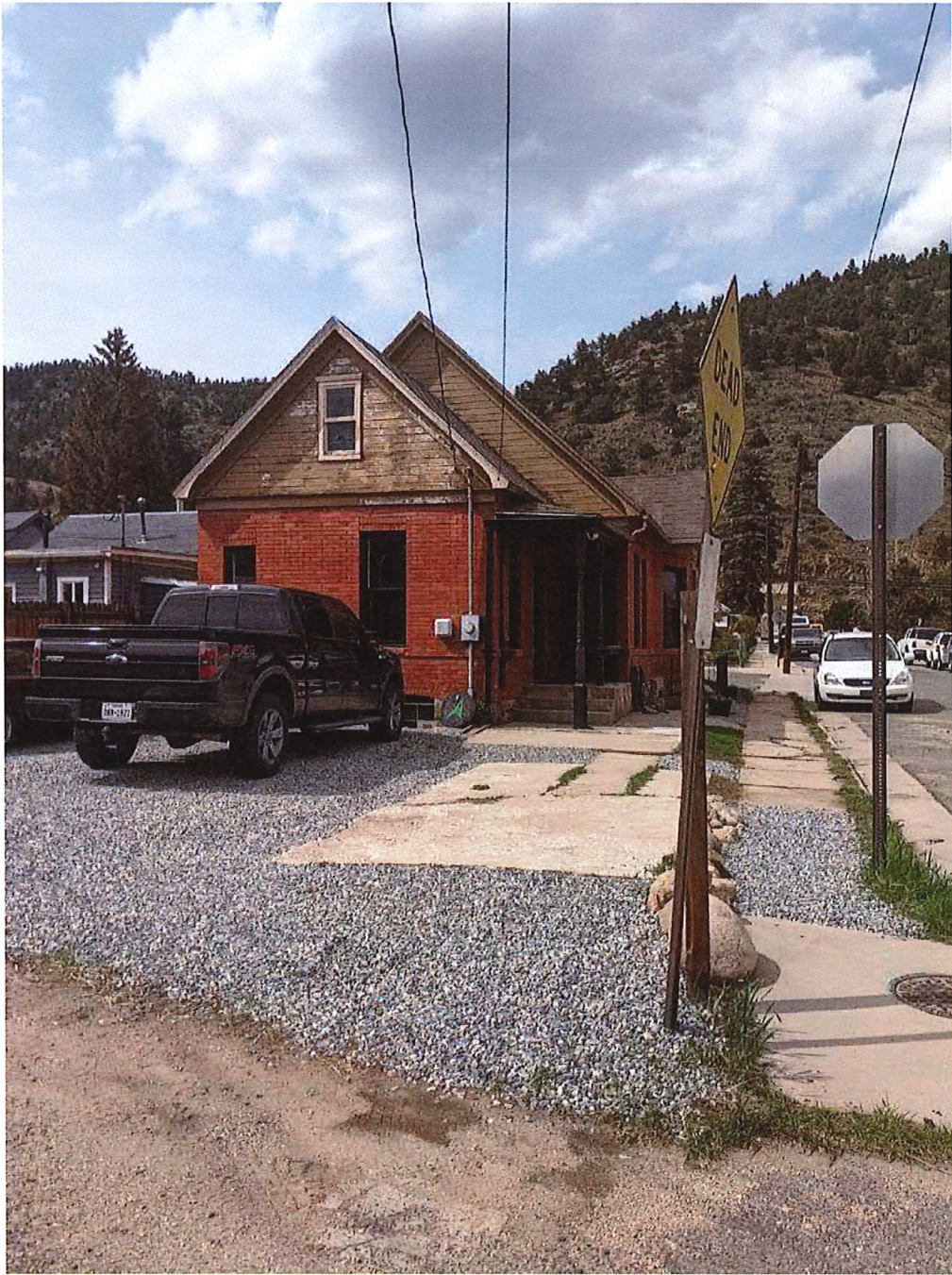
Existing Condition of the parking area.
