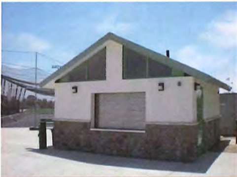
Small Restroom/Concession (~300 SF)
