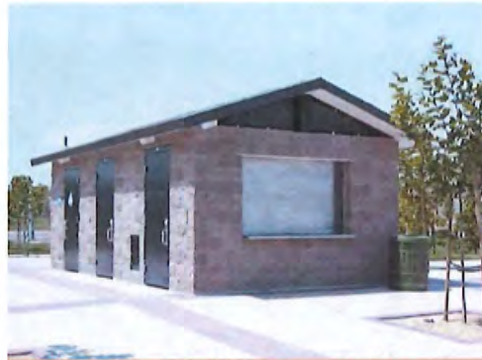
Small Restroom/Concession (~320 SF)
