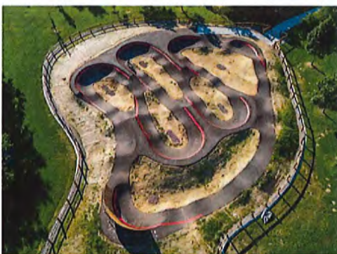
Montebello Pump Track Denver, CO (~14,000 SF)
