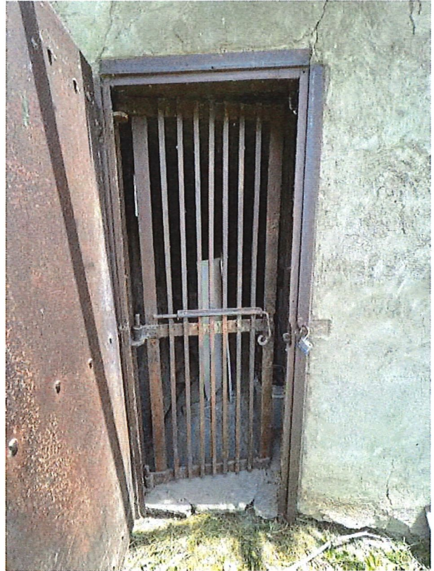
Interior Door for viewing into Powder House
