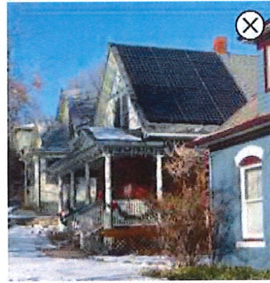
39. On a side-facing roof plane of a primary structure, minimize visual impacts by locating solar collectors at least 3 feet back from the front eave. The collectors illustrated above are not setback 3 feet.
