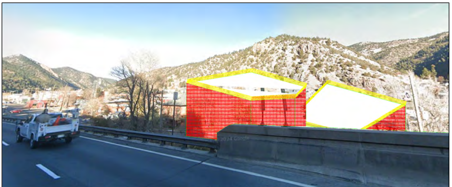
Viewed from I-70 looking north.
