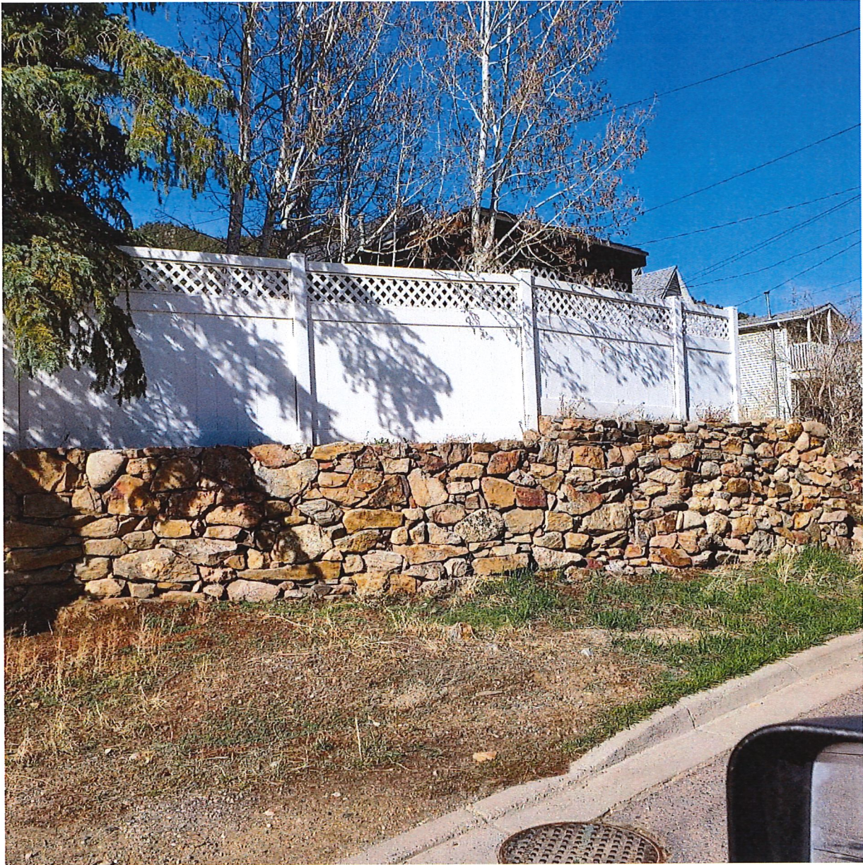
Existing south side of rear yard
