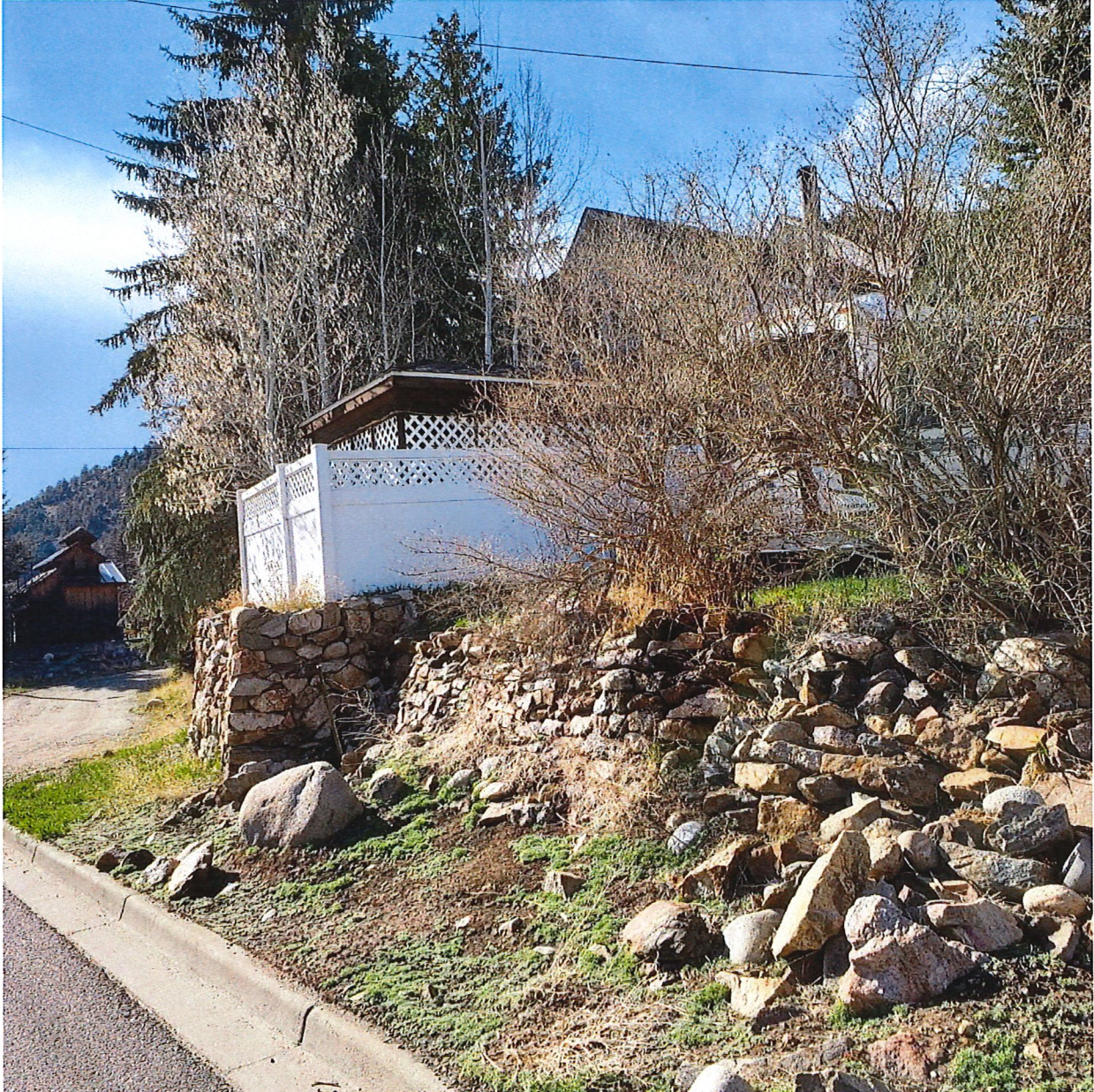
Existing east side of rear yard
