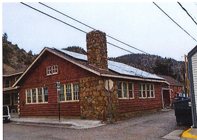
Rear addition at the alley
