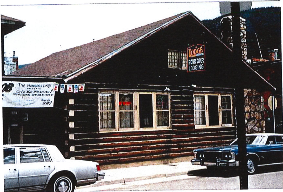
West Facing Side Southern Portion of Hanson's Lodge, Idaho Springs, Colorado, Summer 1997.
