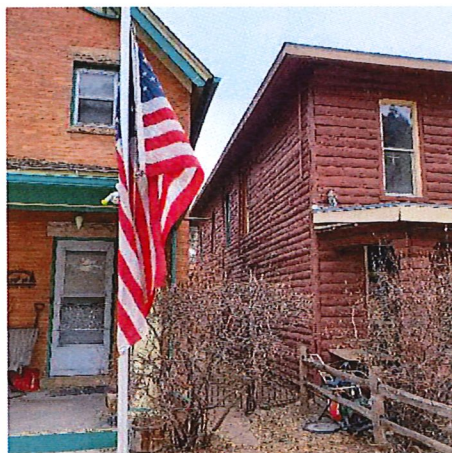
View along east side property line Hi Lana,
