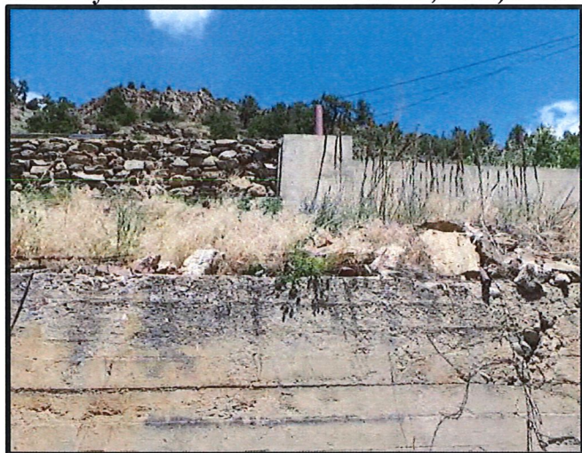
Close-up of retaining walls behind mobile homes.
