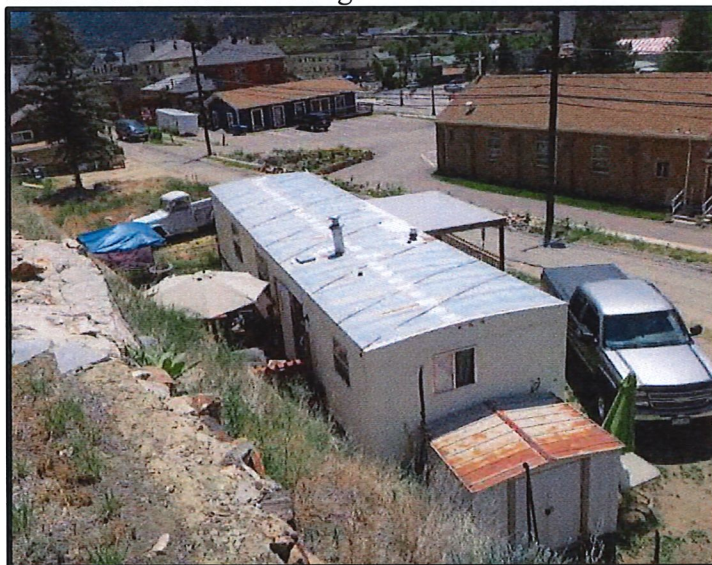
Roof of Cullen Mobile Home with adjacent shed.
