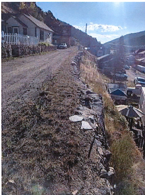
Stacked Stone retaining wall supported by wire mesh
