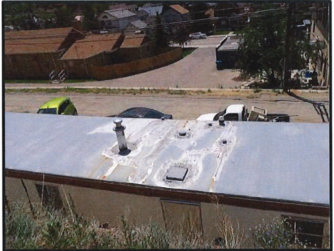
Roof of Eddings / Ruschmyer Mobile Home.
