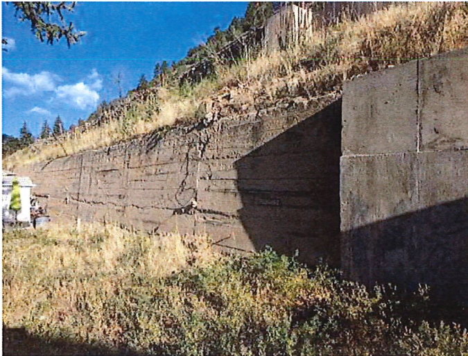
Concrete retaining wall in question.
