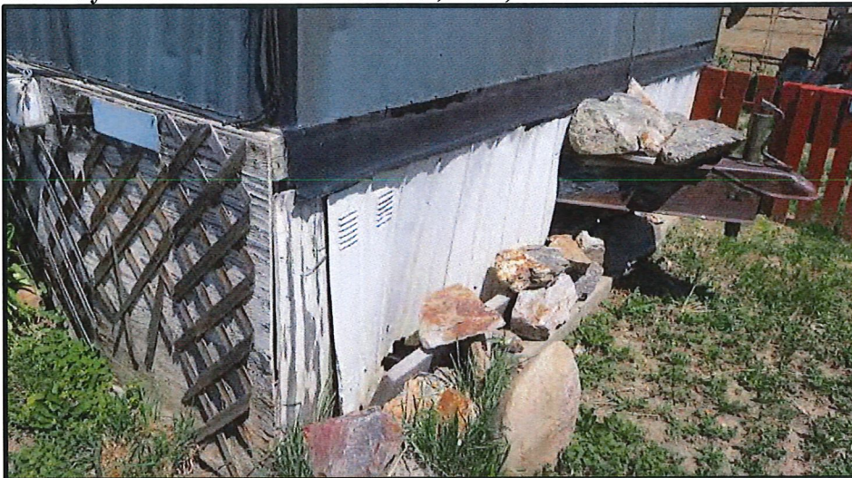
East end of Cullen Mobile Home—Plywood "Skirt" and Rock Foundation.
