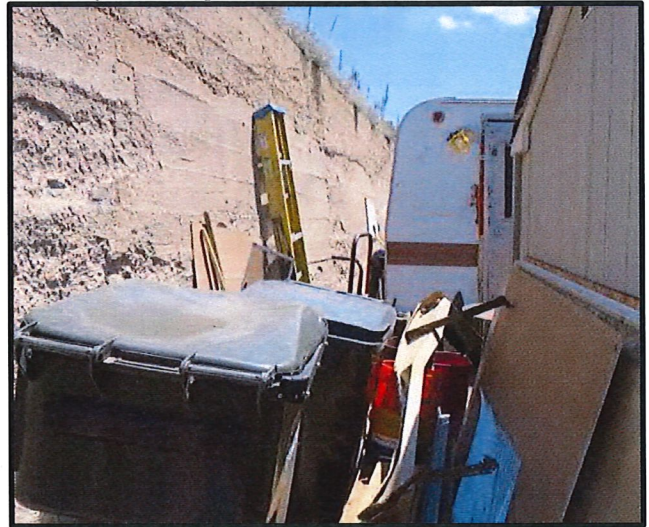
Wall behind Eddings / Ruschmyer Home looking E.
