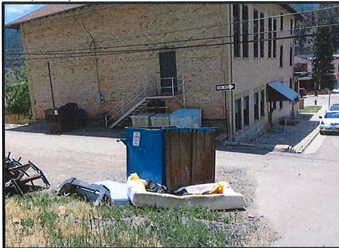
Looking South (BPOE Bldg) from SW corner.
