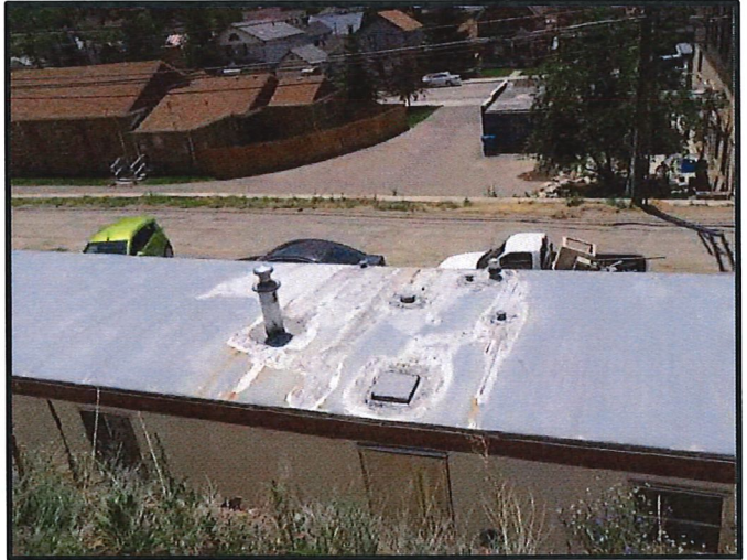
Roof of Eddings / Ruschmyer Mobile Home.
