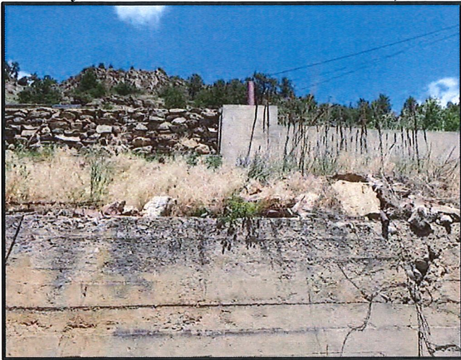
Close-up of retaining walls behind mobile homes.
