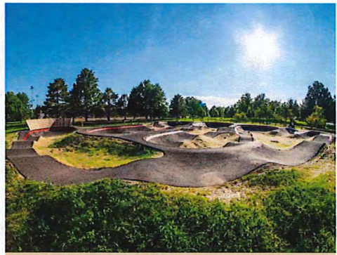
Montebello Pump Track Denver, CO (~14,000 SF)
