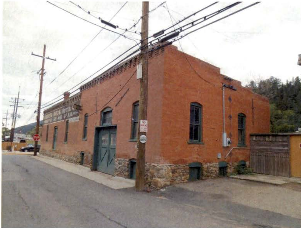
Photo 3: 121 15 th Avenue. View to southeast.
