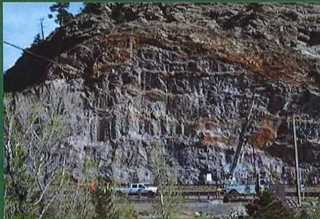
Existing Rock Cut North of Westbound I-70, East of Veterans Memorial Tunnels
