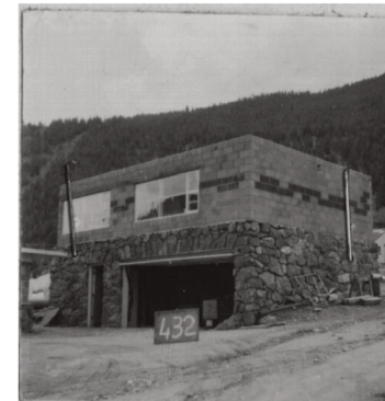
Block D as it appeared in 1949. Note that at this time it is not connected to the main building. The window on the left is now fully covered in siding, and the lower half of the center window is covered. The garage door has been infilled. (Clear Creek County Assessor Card, 1949).
