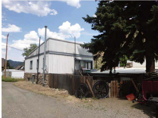
Photo 1: 2815 Miner Street. Block D. View to northwest.
