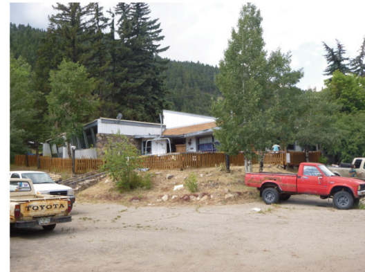
Photo 4: 2815 Miner Street. Block B is partially visible in this image (on left). Note the angled wall on the left side of the photo. The original butterfly roofline is visible in this photo. The fascia board just below the shingle roof shows the original angle of the roofline on Block A. View to southwest.
