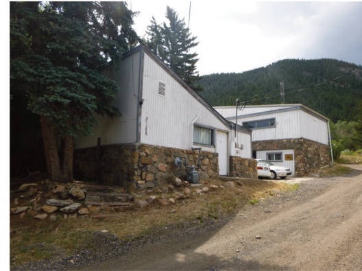
Photo 3: 2815 Miner Street. Block C in front, and Block D in rear. View to south.
