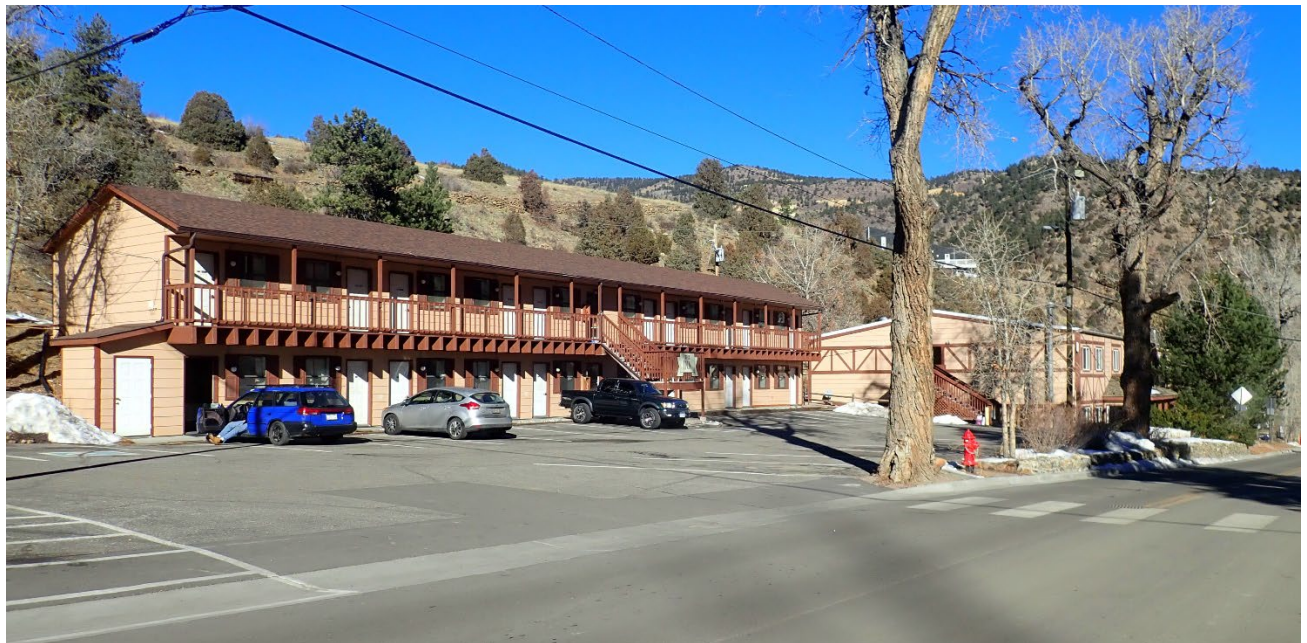
Photo 6: Building 2 in foreground and Building 3 in background. East and south elevations, view northwest. 2020.
