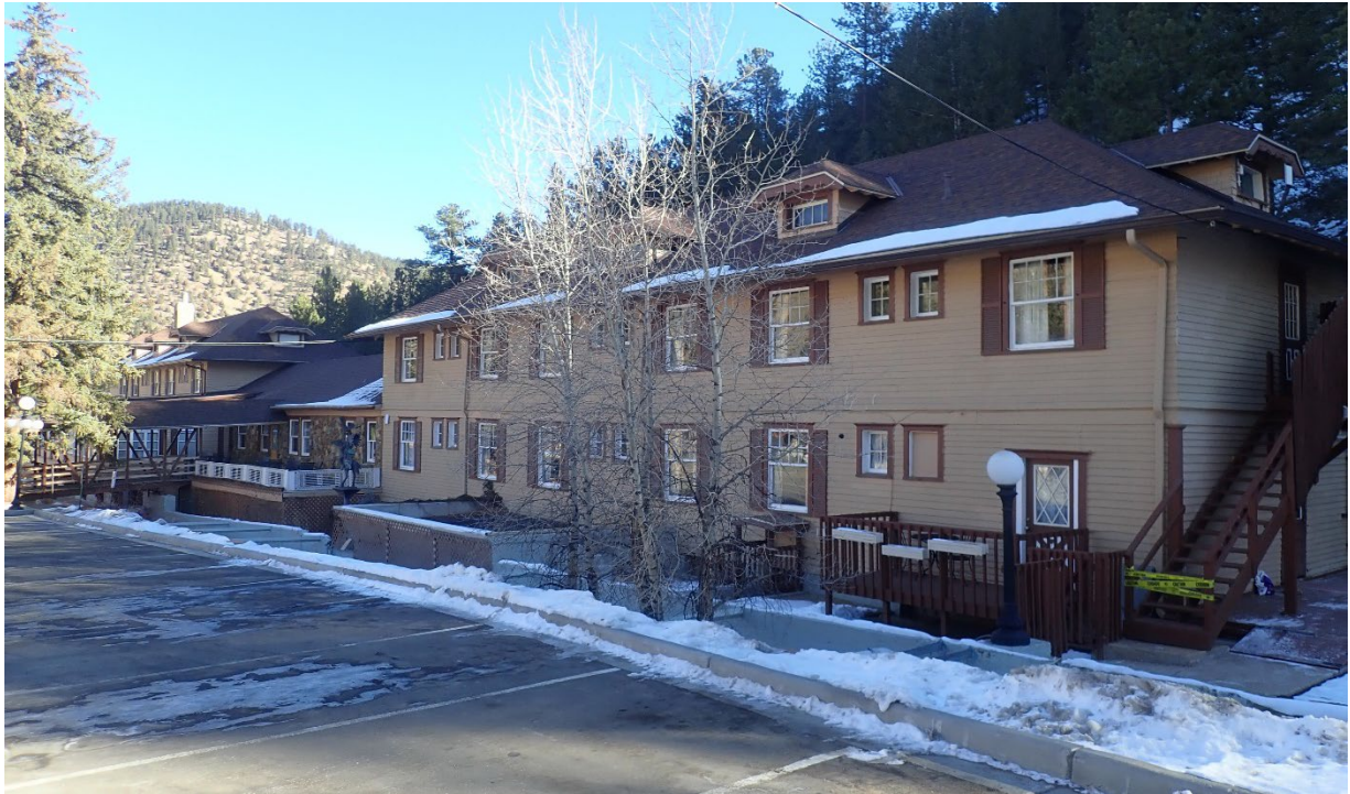
Photo 1: Primary building Block 4 in foreground. West elevation, view northeast. 2020.
