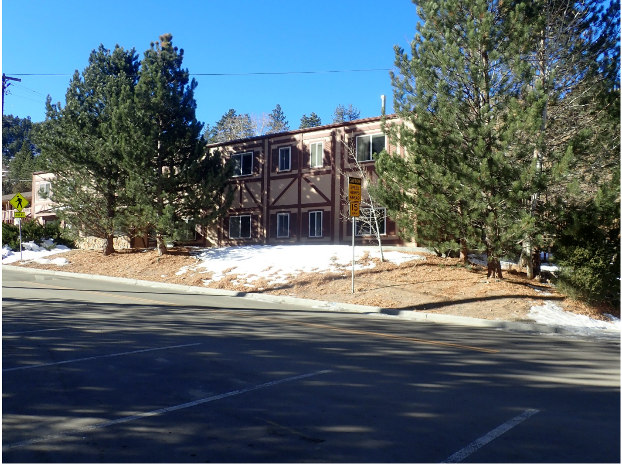
Photo 7: Building 3. East elevation, view northwest. 2020.
