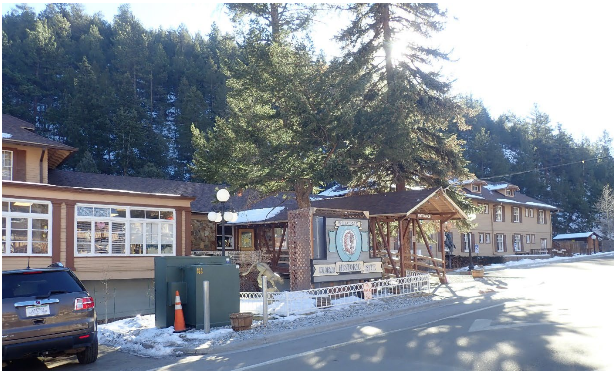
Photo 3: Primary building, from center. West elevation, view southeast. 2020.
