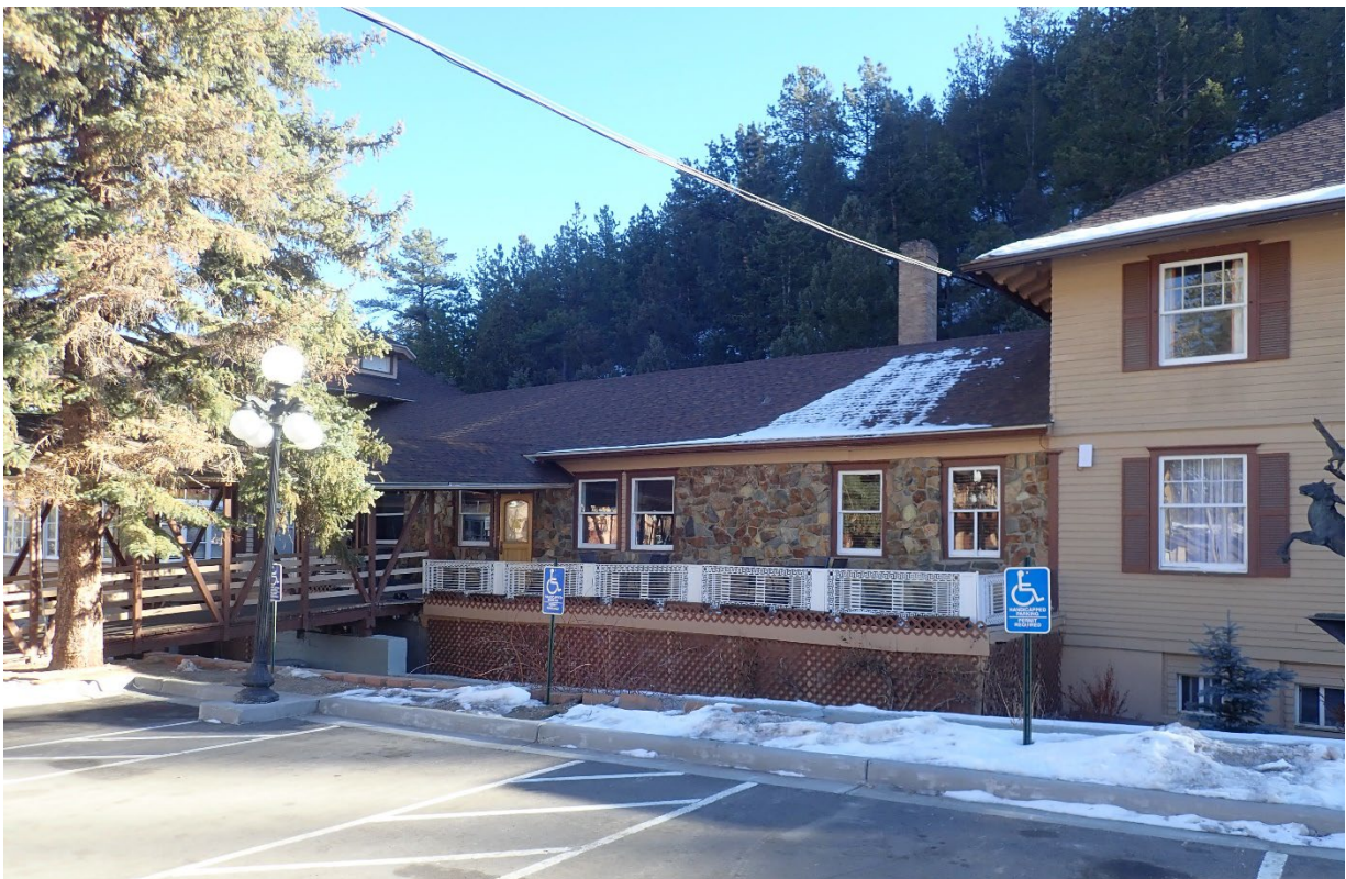
Photo 2: Primary building, Block 3. West elevation, view northeast. 2020.
