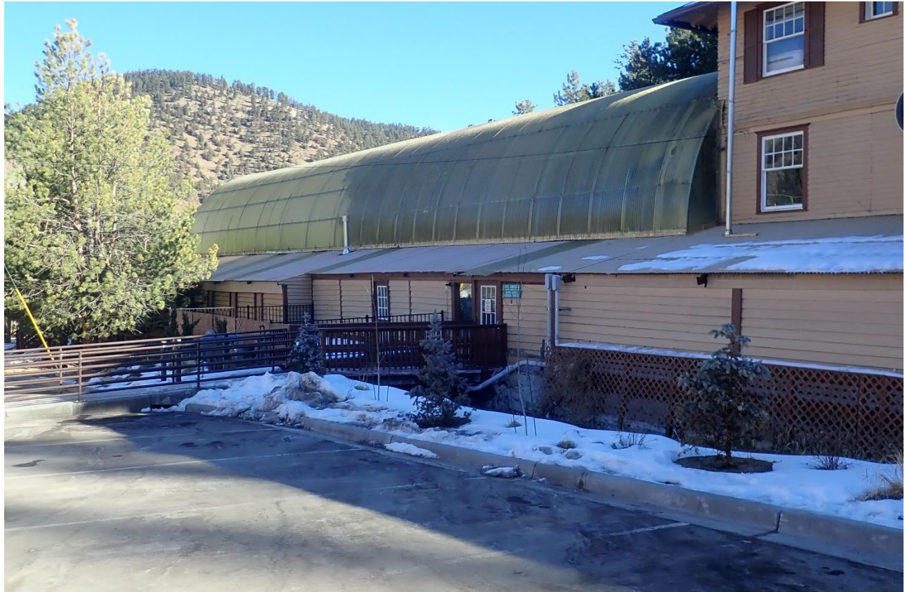
Photo 5: Primary building, Block 1. West elevation, view northeast. 2020.
