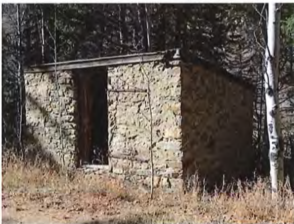
Figure III-8. Large stone rubble was utilized at the building corners. It appears similar to quoins and serves both a functional and decorative purpose for this utilitarian building.
