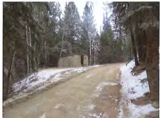
Figure IV-1. The powder house is located along a dirt road off Little Bear Creek Road. Parking spaces could be provided near the main road, thereby preventing cars from being in close proximity to the historic building and retaining the historic character of the site.
