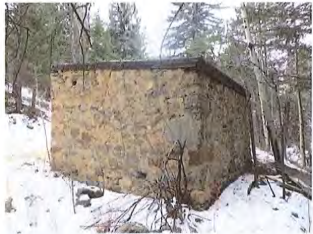
Figure III-2. The west side of the powder house slopes down to Soda Creek, although grade is not level along the west wall.
