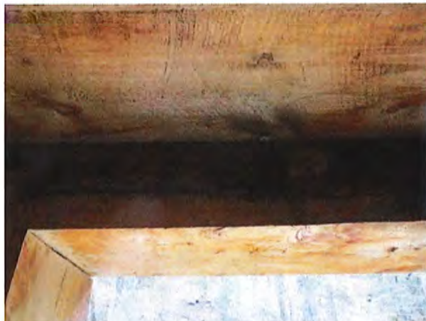
Figure III-23. The head of the door frame is in good condition. Stone rubble was laid in a void above the frame.
