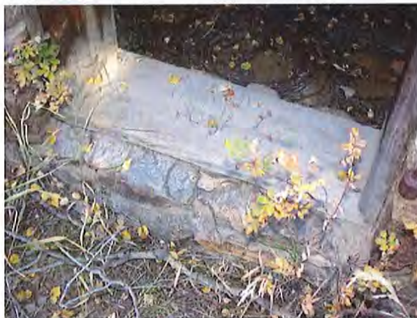
Figure III-18. The original wood threshold remains intact. It was installed on a short section of the stone rubble wall and is raised above grade.
