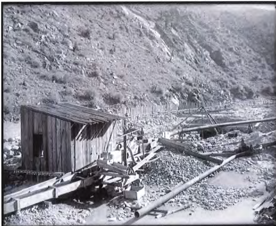
Figure II-5. A hydraulic hose and sluice box are seen in this placer mining operation between 1890 and 1910 along the banks of Clear Creek. Illustrations like this one could be displayed on a plaque near the powder house. (Photo MCC-374 courtesy of Denver Public Library Western History Department)
