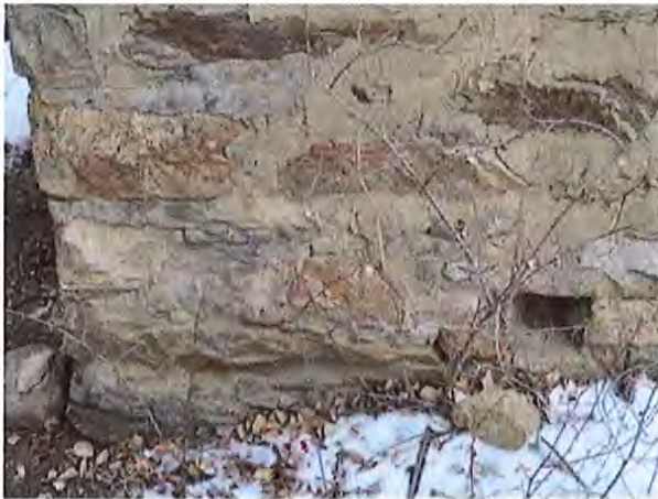
Figure III-28. The south wall incorporates two small openings for ventilation. This one is located near the southwest corner of the powder house.
