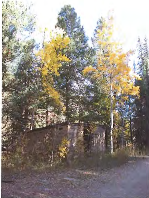
Figure III-3. Shrubs, saplings, and weeds are growing near the powder house.
