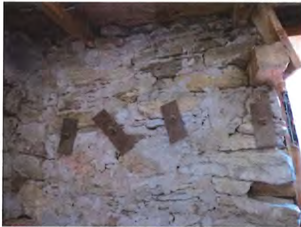
Figure III-20. Although the entry door is missing, it is apparent that it was heavy, given the length of the strap hinges and their attachment with steel plates to the interior side of the wall.
