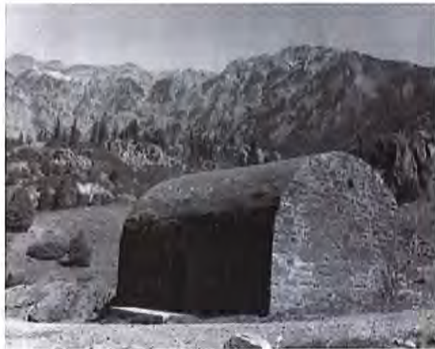
Figure III-3. The stone rubble Revenue Powder House is unique with its vaulted roof. It is located south of Ouray, Colorado. (Photo courtesy of Denver Public Library Western History Department)
