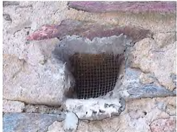
Figure III-29. The ventilation openings incorporate welded wire mesh screens.
