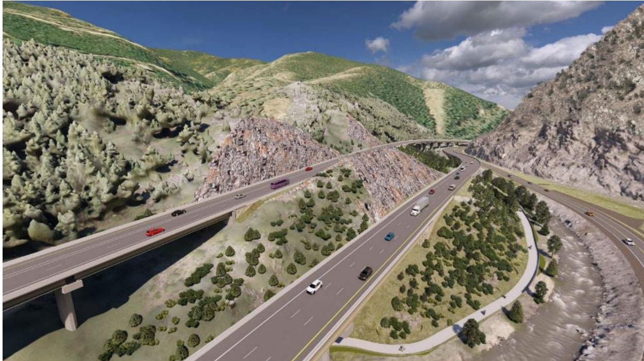
Figure 5. Vertical alignment of I-70 through the “saddle cut” lowers the elevated eastbound section compared to the EA Preferred Alternative
