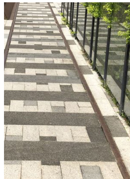
Rail / Track Paving Inlay
