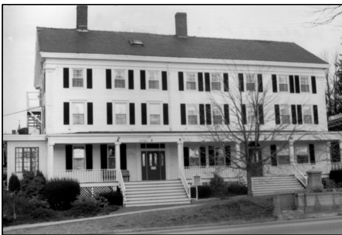
Tavern after rehabilitation before appropriate entrance installed.
