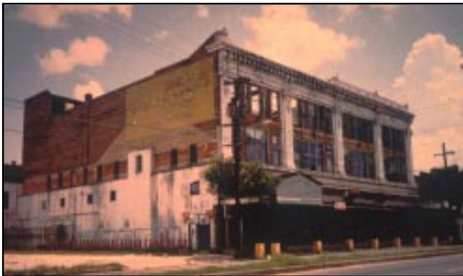
The side elevation of a 1914 department store featured several non-historic openings which had been added over the years.
