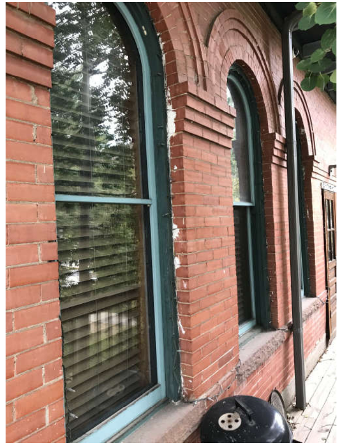
Figure 4. Both fixed and operable windows were provided circa 1986. The fixed window is in the foreground; the operable one is beyond.
