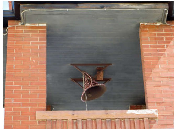
Figure 7. Proposed work at the belfry includes preserving the beaded board ceiling and cast iron bell assembly.
