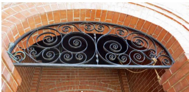
Figure 6. The original ornamental metal grille at the front entry will be preserved with this project.
