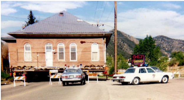
Figures 1 & 2 (Above & Below). View of schoolhouse being moved down Miner Street. (Source: Historical Society of Idaho Springs)
