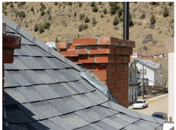
2. Existing surface-applied counterflashing at belfry.
