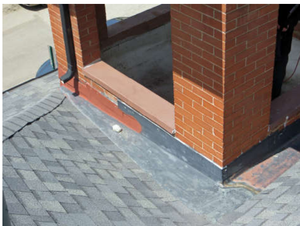
3. Existing surface-applied counterflashing at belfry.
