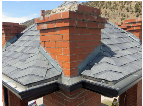
1. Existing surface-applied counterflashing at belfry.
