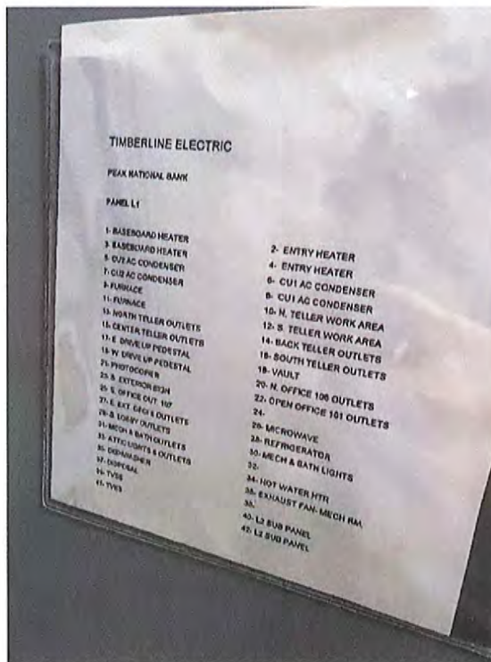
Figure 17: Existing panel schedule for Panel L1
