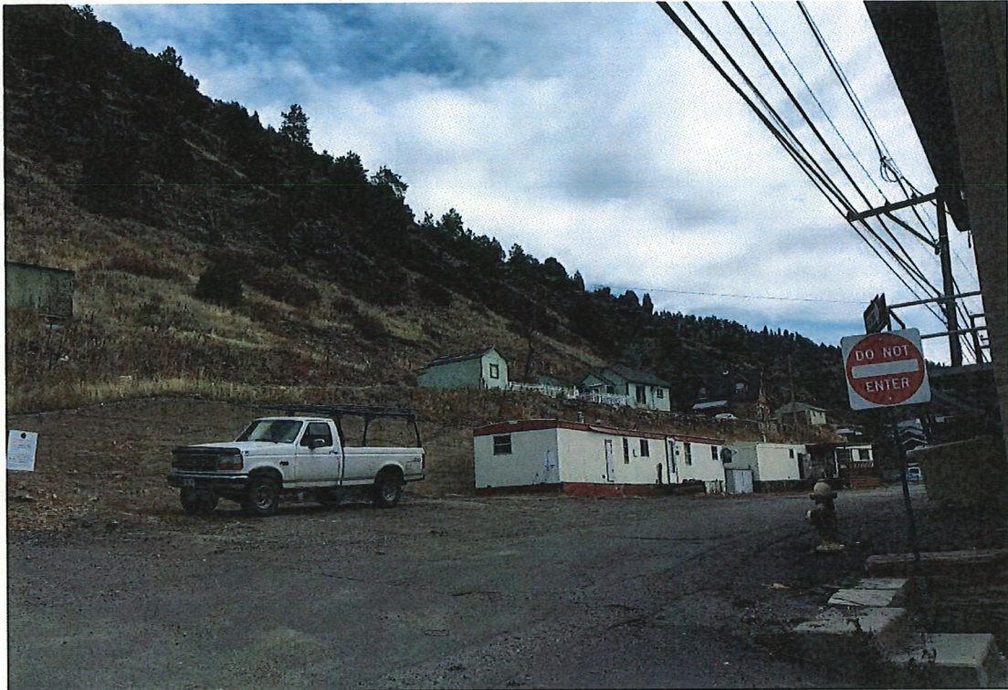
Subject property and retaining wall looking east.
