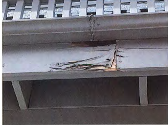
South side (Miner Street) of veranda
