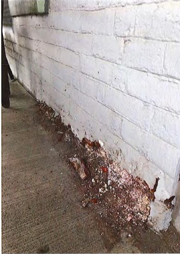
South wall (Miner Street) under the veranda
