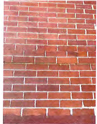
Repointing mortar joints ensures that brick construction is preserved long-term
